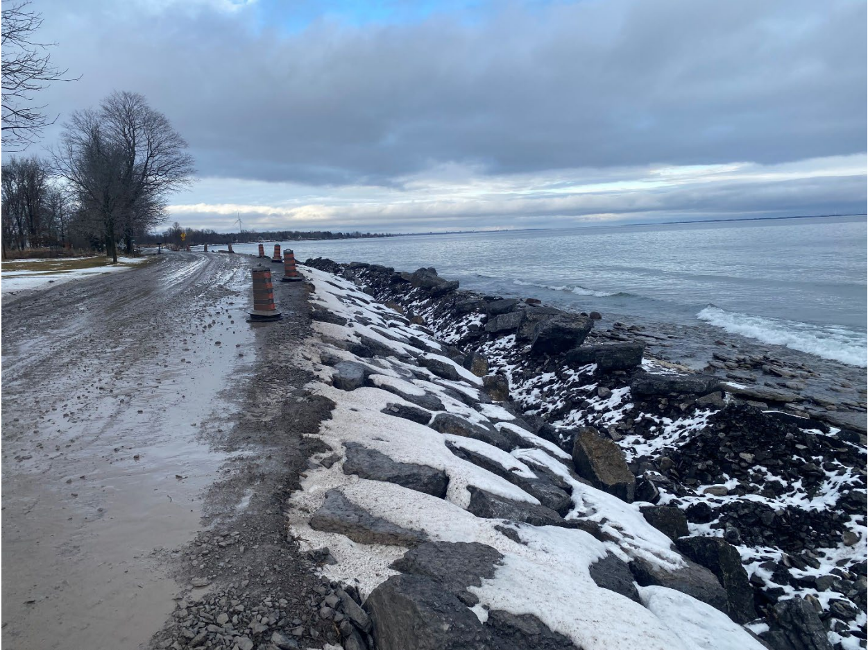
Figure 1 Shoreline protection project, South Shore Road - January 2023
